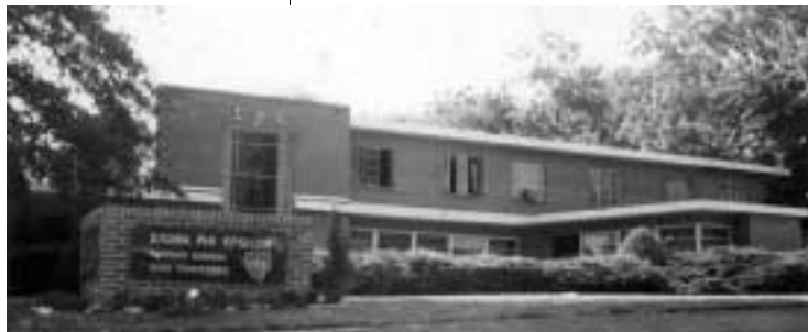
KS GAMMA CHAPTER HOUSE AS IT WAS CONSTRUCTED IN 1949
