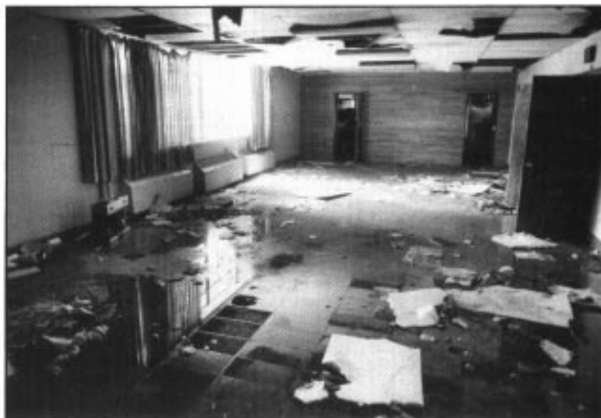
The Dining Room shows signs of extensive water damage. Although the fire was contained on the upper level, the entire first floor was damaged by smoke and water. The fire restoration work replaced all ceilings, furnishings, and window, wall, and floor coverings. In addition, the Alumni Board had the wall at the right removed for an expansion of the Library into the Dining Room.
