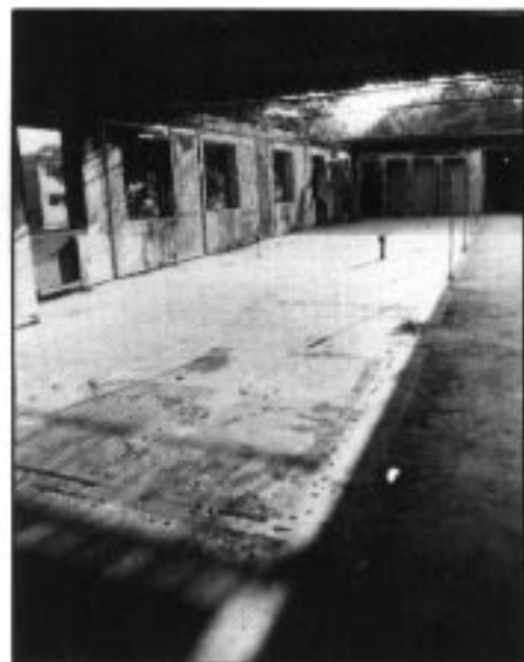
Above: As the demolition work is completed inside the Sig Ep "shell," one could see this view looking west from the top of the main staircase. The president's room, No. 1, was in the area in the immediate foreground. Note that part of the roof structure has been removed.
